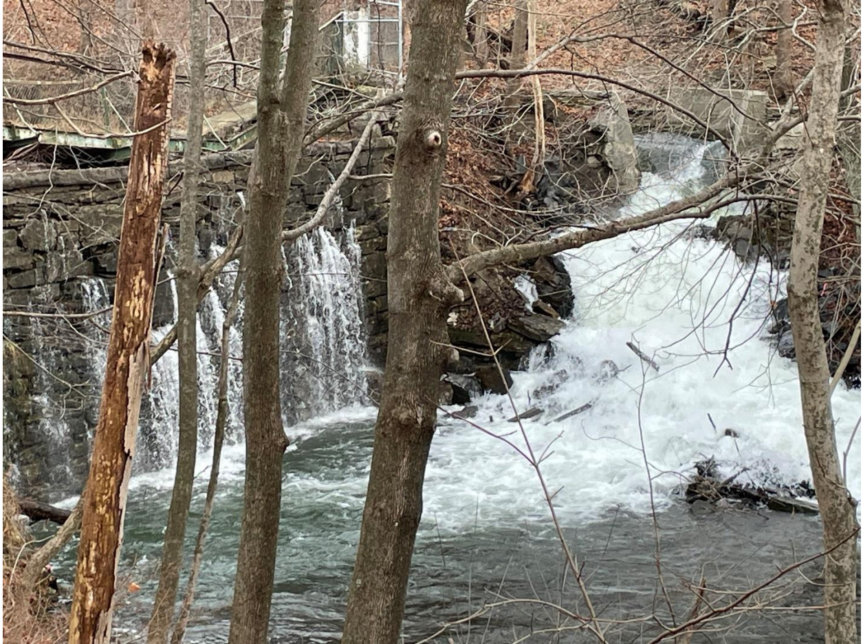
Figure 9: Heavy water flow from spillway and leaks in dam visible at time of visit, facing north east (12/19/23).
